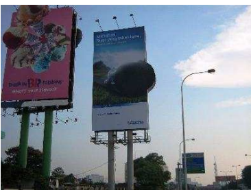
Dowble Sided Twin Pole Vertical 60' x 30'
